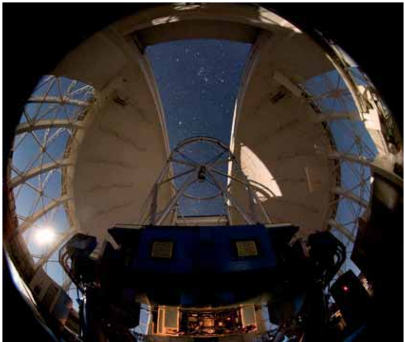
Figure 2. View of the Gemini South dome (from inside) and telescope. The Near-Infrared Coronagraphic Imager (NICI) is the instrument visible attached to the Cassegrain instrument support structure. Three other instruments (not visible) are mounted on the remaining ports.
